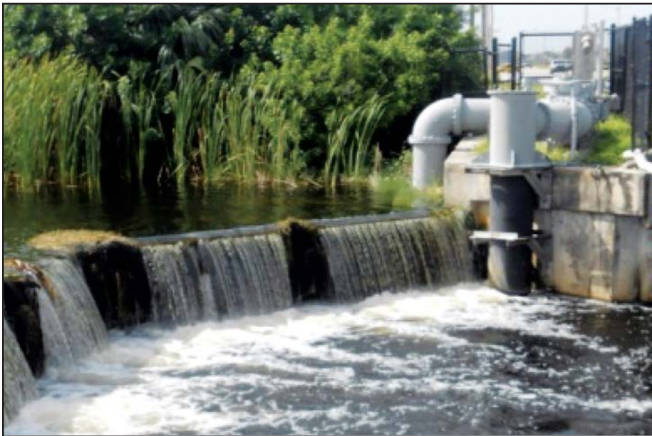
Figure 11. Stormwater harvesting for irrigation in Cape Coral.
